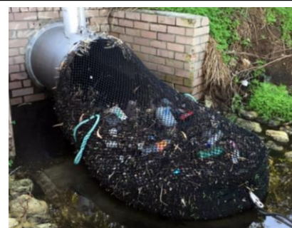
A drain sock is a simple solution to the problem of stormwater pollution.
